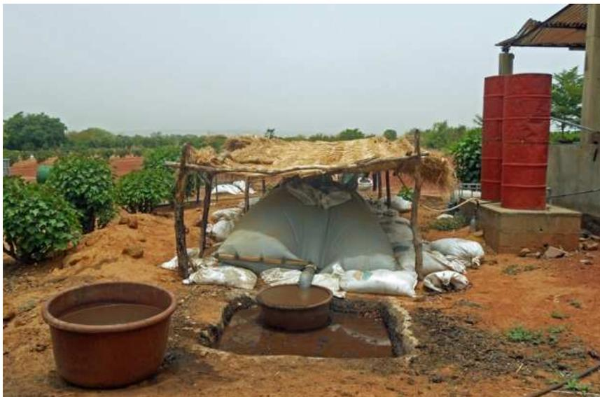
**Figure 2: A bag-type anaerobic digestion system, as implemented in Koulikoro, Mali (Mali\_Biocarburant 2012)**
